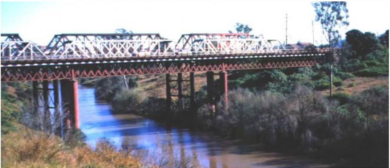
The three Bremer River rail bridges in 1964. The original bridge is in the foreground then the second bridge (with the silver trusses) and the final bridge in the background.
